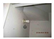
The closet wall or ceiling has moisture damage and stains and needs to be evaluated and repaired as needed.
