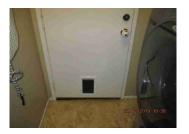
The fire-rating of the house entry door has been nullified by the addition of an animal door it will need to be replaced.
